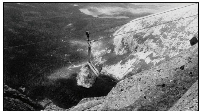
Boulder going down the line under belay
