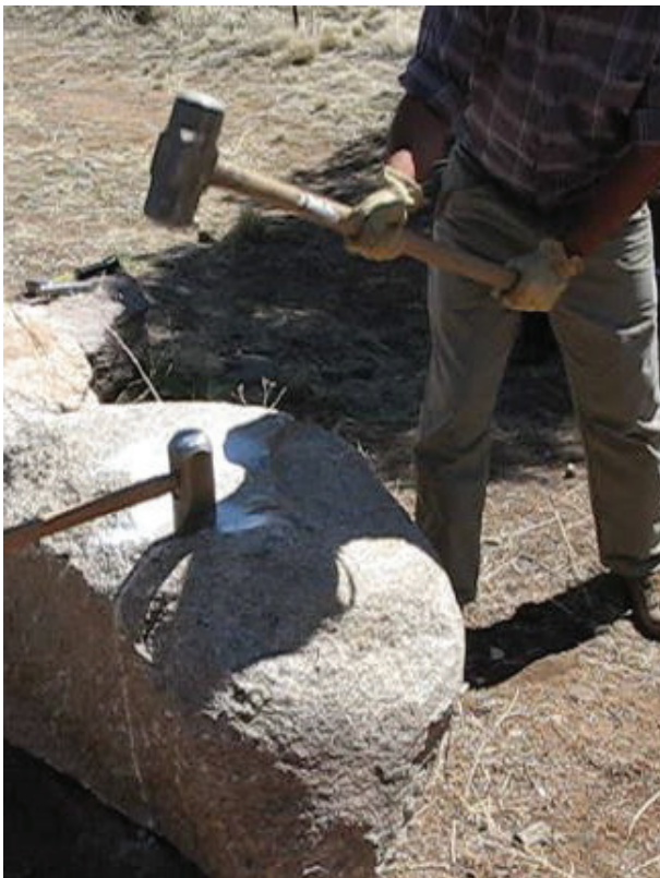
Scoring Stone with rifting hammer and sledge. Arizona Trails Association, Prescott AZ, 2009
