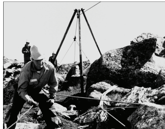
Rope belay controls descent of boulder
