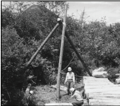
18 ft. tall tripod supports high line.
