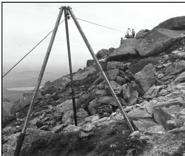
Black extensions level tower on side slope
