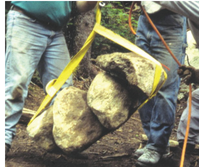
4 boulders in a B4 custom sling.
